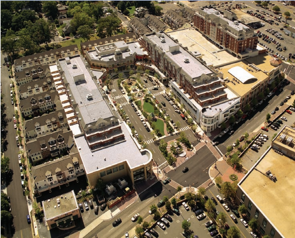
The development of the Market Common, Clarendon in Arlington, Virginia, included enveloping this mixed-use development with townhouses that increased density and shielded the surrounding neighborhood from back views of the shopping center.
