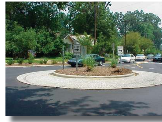
Roundabouts allow vehicles, including bicycles, to continue moving, although at reduced speeds.
