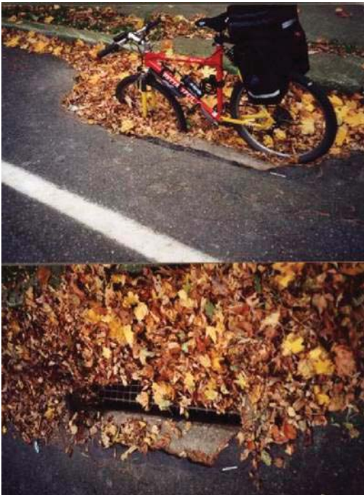
These images show the importance of well-designed drainage grates.
