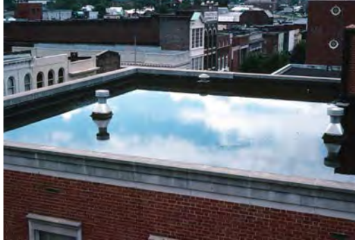
Blue roofs detain stormwater
