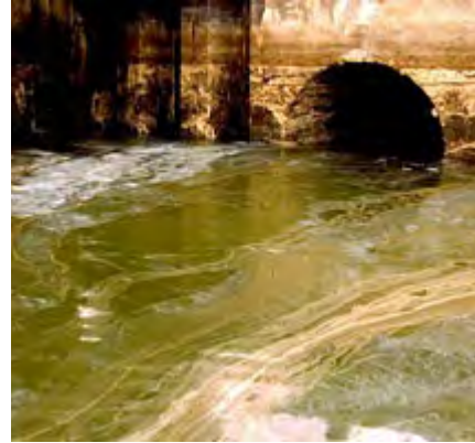
Combined sanitary/stormwater sewer outfall
