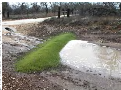
Example of compost filter berm to prevent downstream contamination
