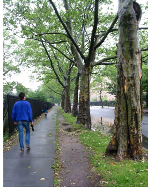
Continuous planted soil trench benefits trees and reduce pavement upheaval
