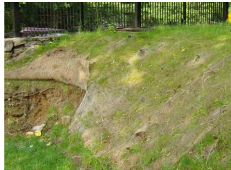
Erosion control fabric and vegetated slope protection at Riverdale Country School
