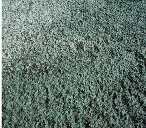
Hydroseeding is a popular technique for applying seeds, fertilizer, and soil stabilizers in a single application
