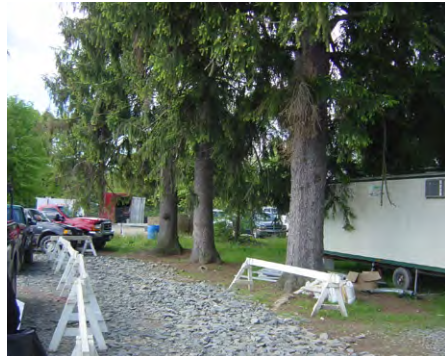
Example of haul road and contractor parking area using gravel over geotextile fabric
