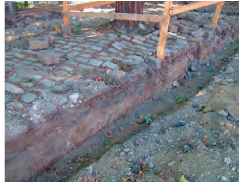
Curb removed from one side protects existing trees
