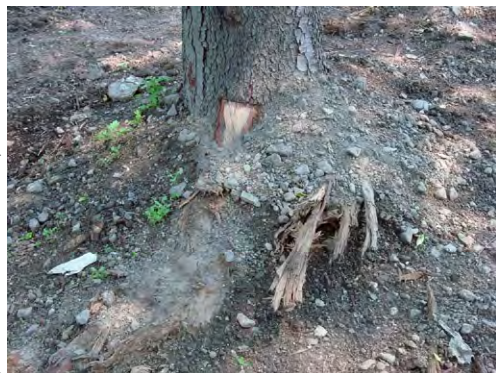
Example of severed structural roots
