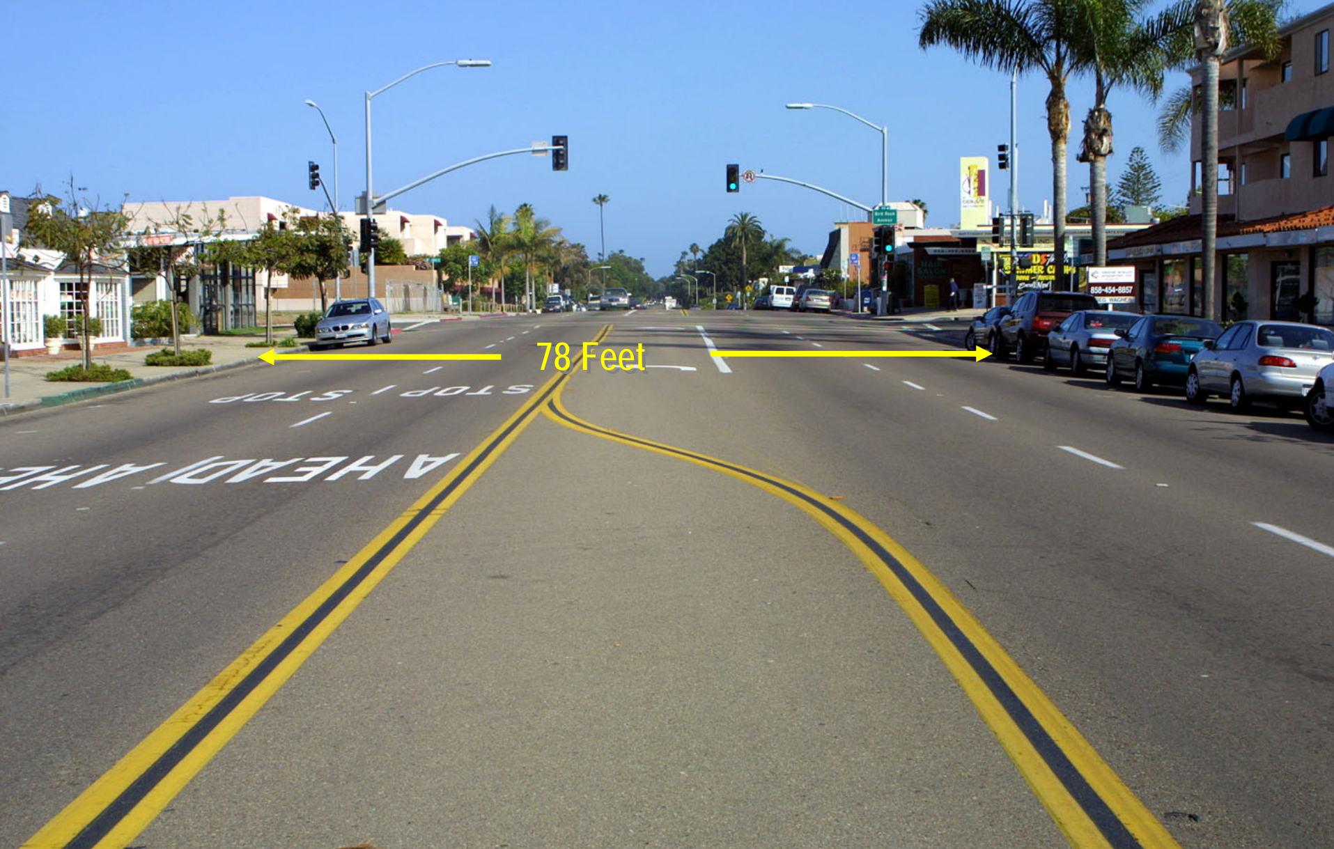
La Jolla Boulevard, Bird Rock, San Diego, California (Five to two lane conversion, before). Four signals and one four-way stop being removed. Back-in Angled parking to be added. (23,000 ADT)
