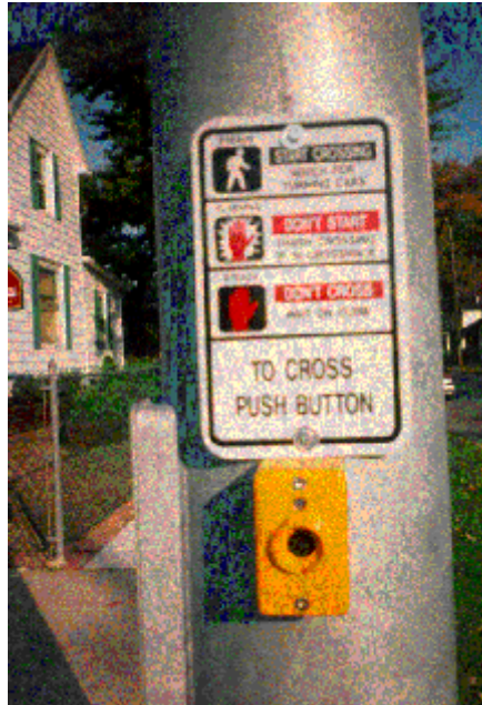
Figure 1. An illuminated push button in Windsor. The orange light is below the button.
